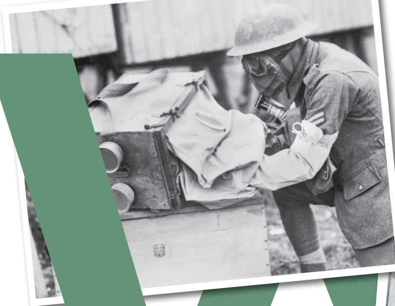
First World War, France, 1918. This gas-proof box was found in a German army pigeon loft. It was used to hold pigeons while messages were being attached to them during a gas attack.
